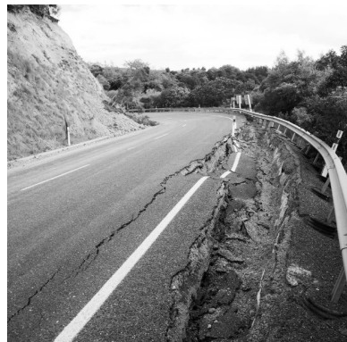
Fig. 9. Road with solid asphalt-concrete coating
