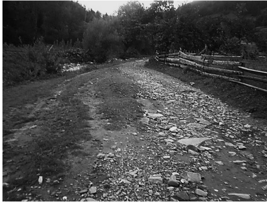
Fig. 3. Use of waste from the stone industry for road pavement
